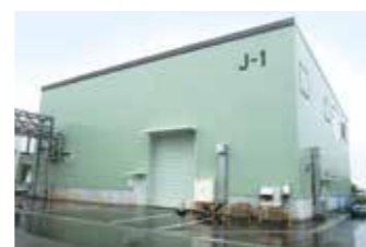
New pure water building at the Koriyama plant
