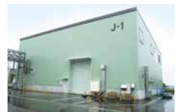
New pure water building at the Koriyama plant
